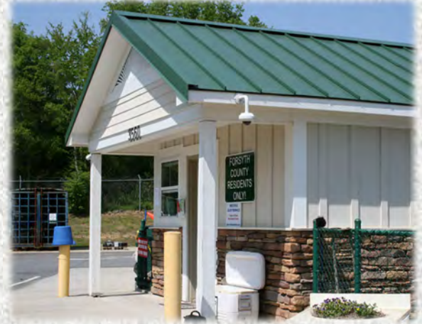
Forsyth County Recycling Center
